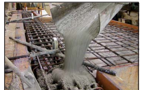
Main characteristics of self-consolidating concrete include: (1) Ability to fill a mold or form; (2) Resistance to segregation (stability); (3) Ability to flow through reinforcing bars or other obstacles without segregation; and (4) Superior surface quality and finishability.
