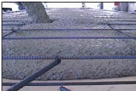
Main characteristics of self-consolidating concrete include: (1) Ability to fill a mold or form; (2) Resistance to segregation (stability); (3) Ability to flow through reinforcing bars or other obstacles without segregation; and (4) Superior surface quality and finishability.
