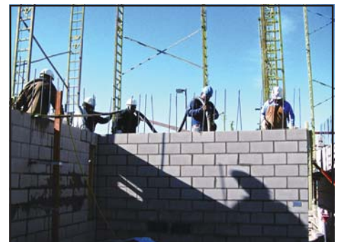
Reinforced masonry with fully grouted cells creates solid confinement for prisoners.
