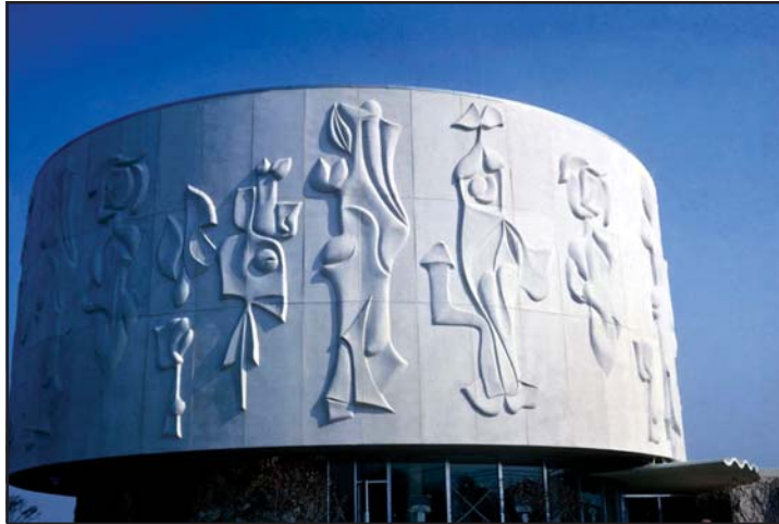
Self-consolidating concrete is able to flow into almost any shape or form, providing excellent surface characteristics. For the Porthaven Professional Building in Cuyahoga, OH, white concrete was used to present the design of sculptor Harvey Wheeler.
