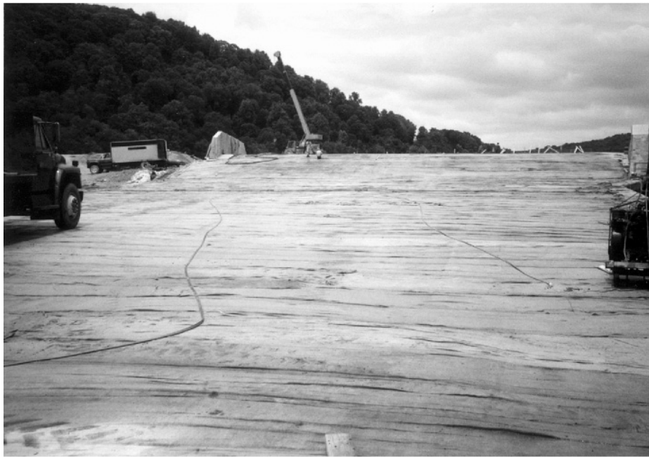
Figure 7. Moist Curing with Burlap (Saltlick Dam Spillway Slab)
