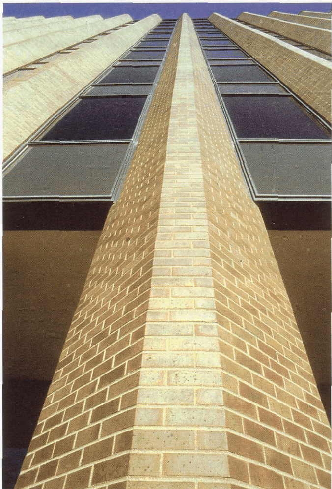
Fig. 6. With care and cooperation, consistent mortar color producing the appearance desired by the owner can be achieved.
