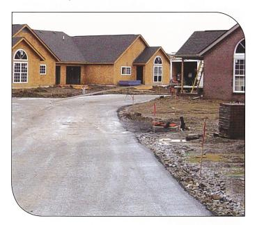
RCC placed during site work serves as a working surface. With a thin overlay, it becomes a residential street once construction is complete.
