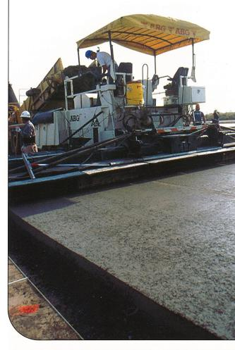
RCC normally is placed with asphalt paving machines; most contractors who specialize in the construction of RCC pavements use high-density pavers with vibrating screeds and oscilating tamping bars.
