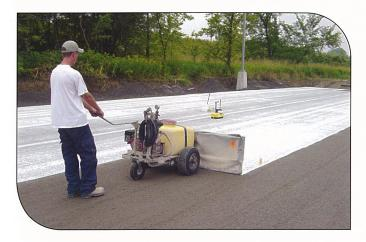
A key to long term performance is adequate curing. Water or concrete curing compounds are typically used.
