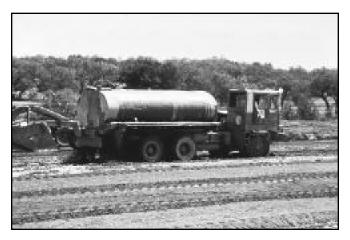
Adding cement in slurry form to clay subgrade for concrete parking lot in Texas.
