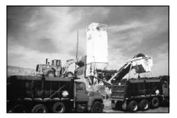
Mixing cement-modified granular material in a central plant for a road subbase in Kansas.
