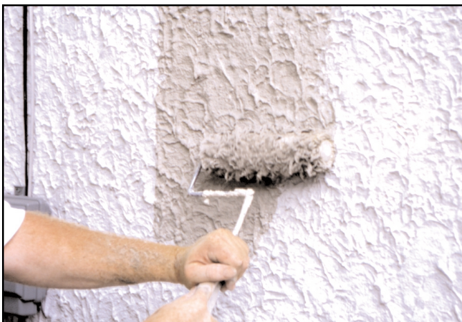
Fig. 10. Coatings provide water repellence, fill narrow cracks, and disguise color differences. (69911)
