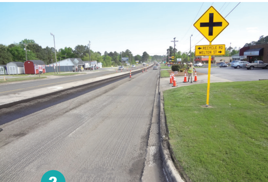
Milling the pavement to lower it two inches below the original gutter elevation
