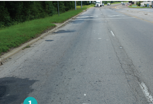
Successive overlays nearly covered the curb while the pavement deteriorated
