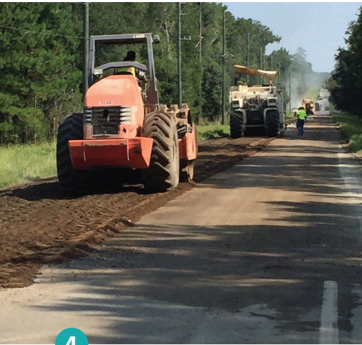
4 Sheepfoot roller compacting FDR
