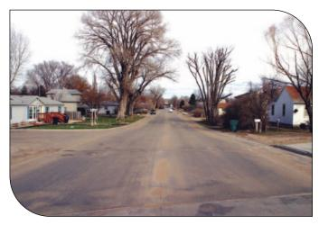
Existing asphalt pavement on West 8th Street had deteriorated too much to accept a traditional ultra-thin whitetopping surface.
