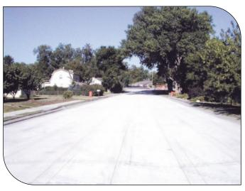
The new concrete roadway provides an economical, smooth, light surface, with excellent strength, durability, and appearance.
