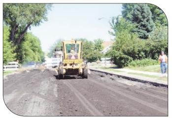
A grader was used to place the new cement-stabilized base, consisting of the pulverized asphalt and old base material.
