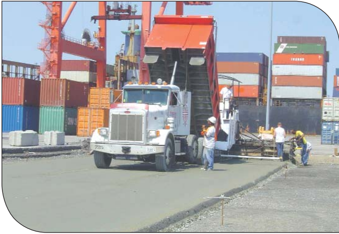
Placing the second lift of the two-lift construction process.
