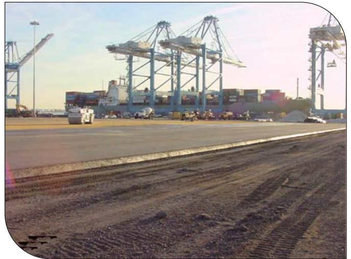
Completed RCC slab at the Port of Virginia.
