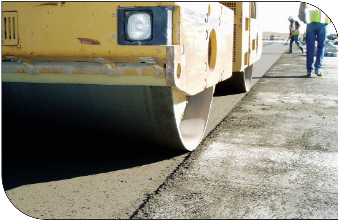
Compaction of adjoining 8-inch (200 mm) RCC layer.
