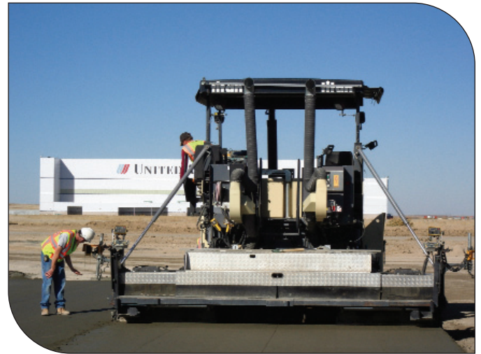
High-density paver placing RCC at DIA.
