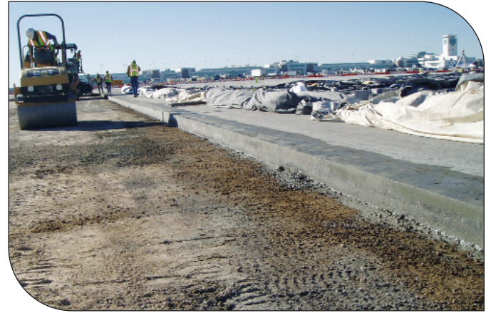
Completed RCC layer showing protective blankets.
