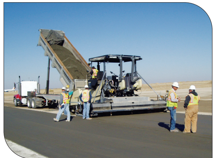
RCC paving operations on snow removal storage area.
