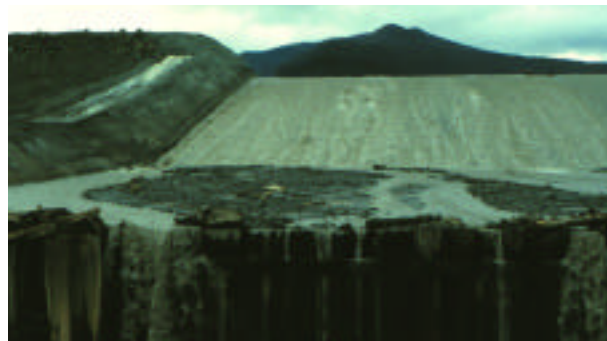
Figure 6. Aftermath of RCC Spillway at North Fork of the Toutle River following 11 months of high velocity flow. Note severe washout behind sheet pile end sill. (S#70046)
