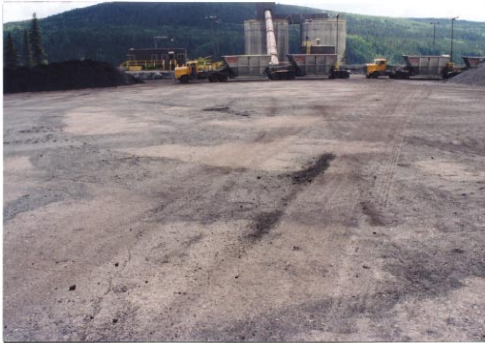
Figure 25 Coal is stored on the RCC surface prior to shipment by rail to offshore markets.
