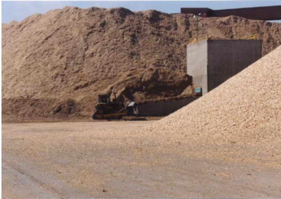
Figure 35 Wood chips are piled to a height of 12 m (40 ft.) on this RCC pavement in Northern Alberta, Canada.
