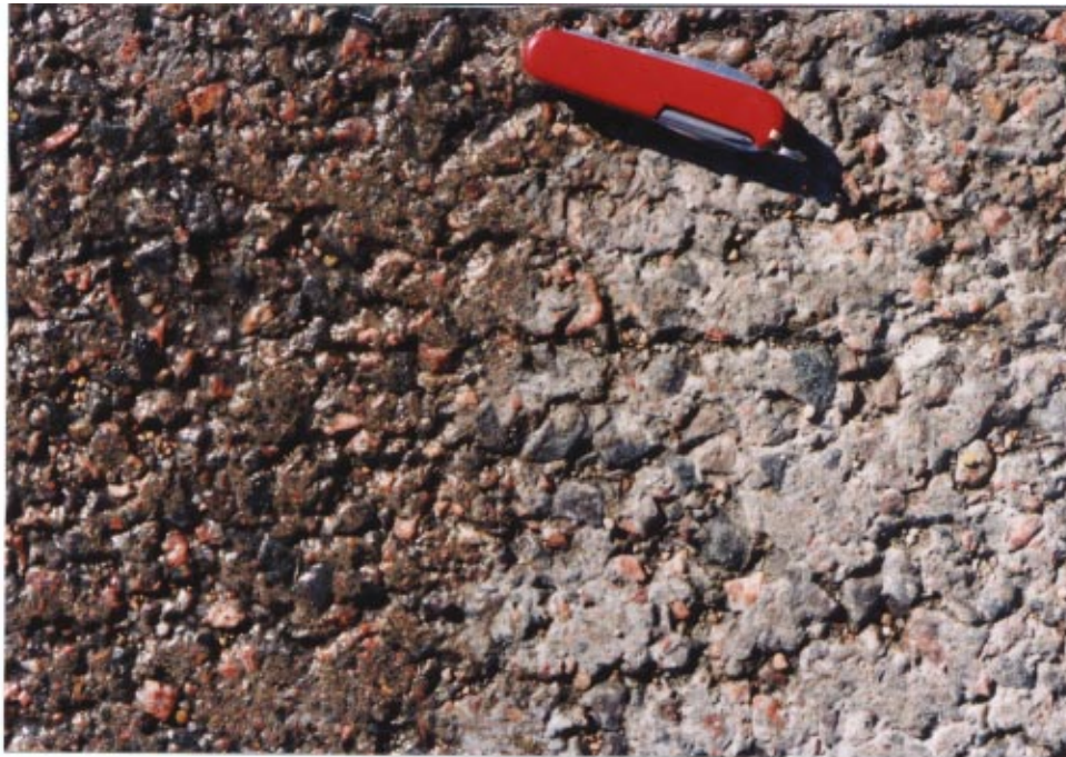
Figure 16 Closeup of the RCC surface. Built 1986.
