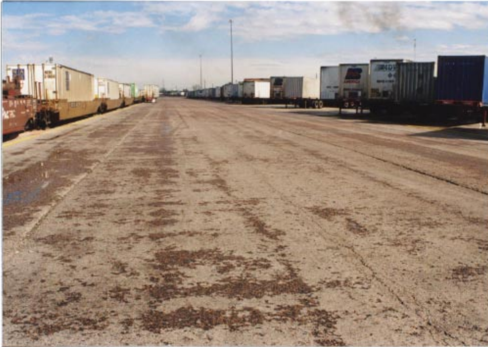
Figure 15 Intermodal Terminal, Burlington Northern Santa Fe RR., Denver, CO
