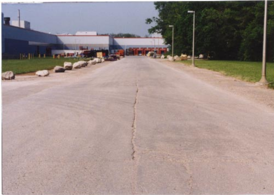
Figure 43 All of the internal plant roads are exposed RCC pavement.
