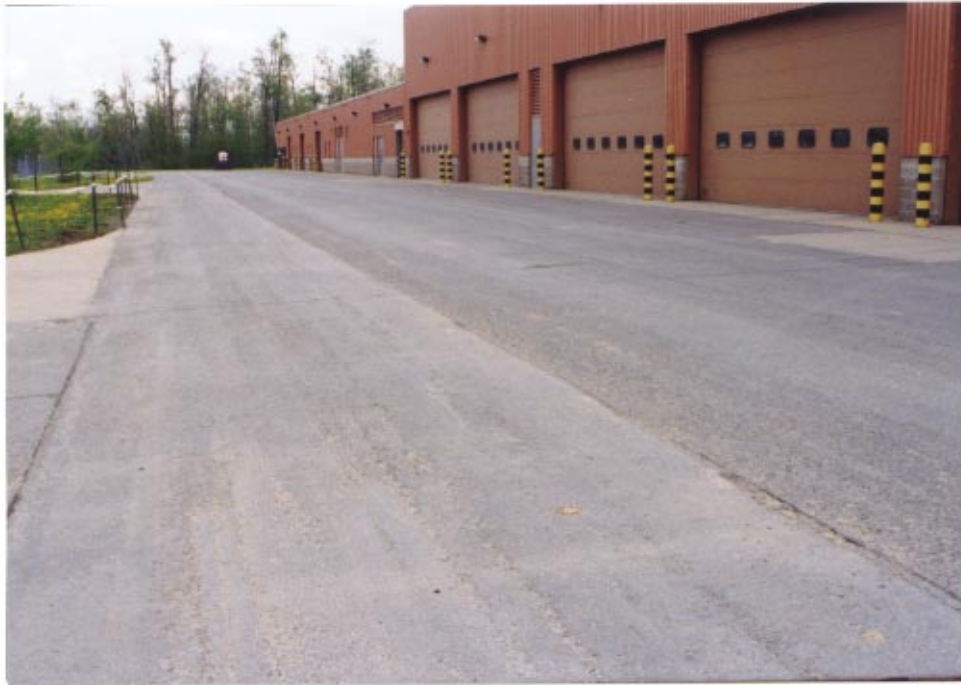
Figure 29 Apron pavement adjacent to an equipment maintenance shop.
