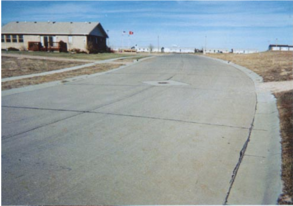
Figure 47 The smoothness of this city street built with RCC is similar to any new pavement built with traditional paving materials.
