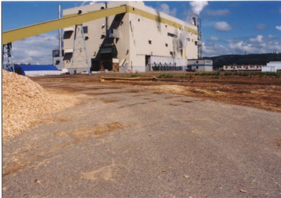
Figure 31 Storage of wood chips on RCC, provides a durable surface that is easy to clean.
