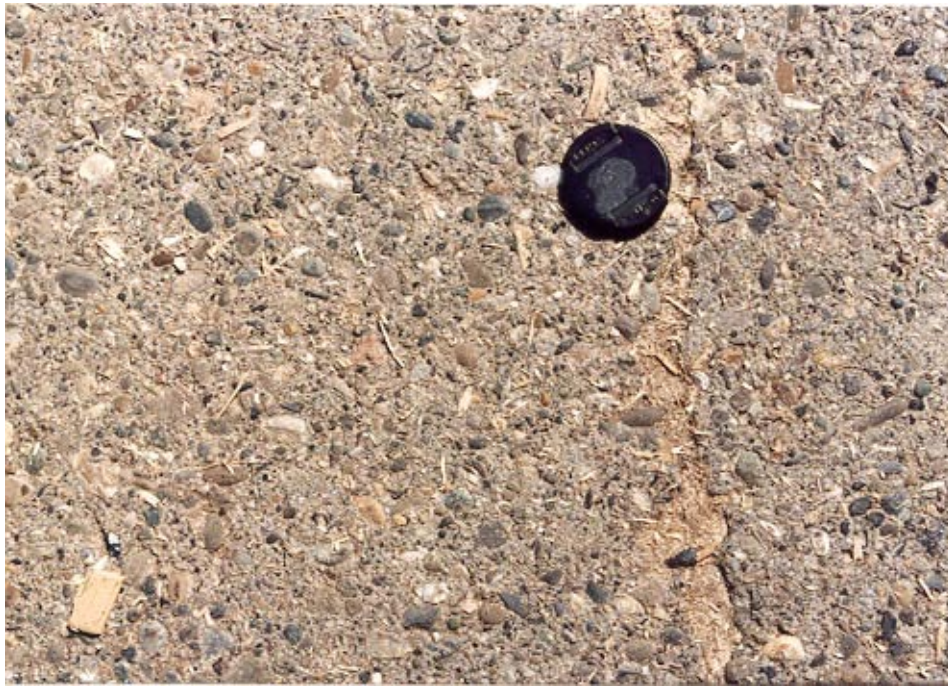
Figure 2 Surface at Fibreco Pulp Inc, Taylor, B.C. Built in 1988.
