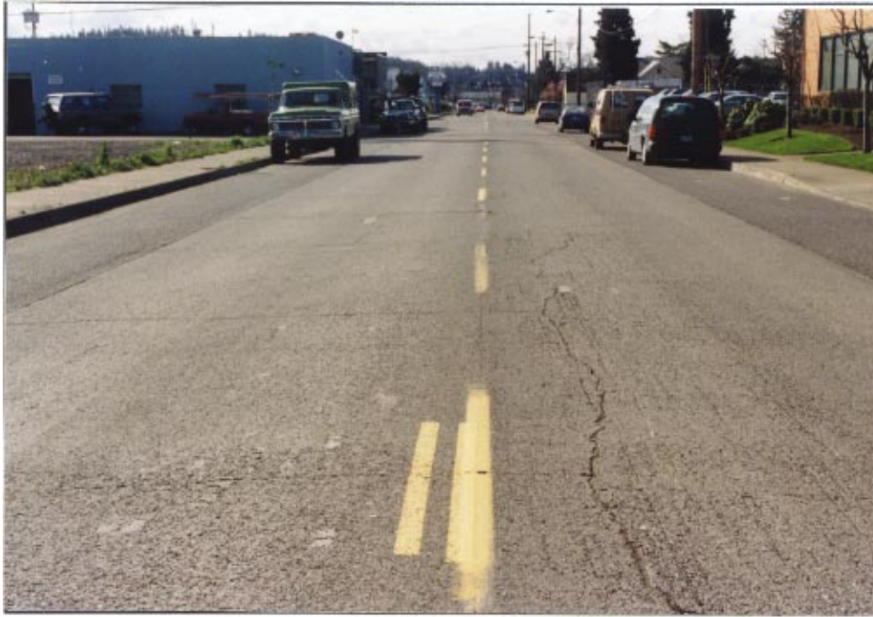
Figure 41 99 th Avenue, Portland, OR. A successful experiment in RCC street paving.
