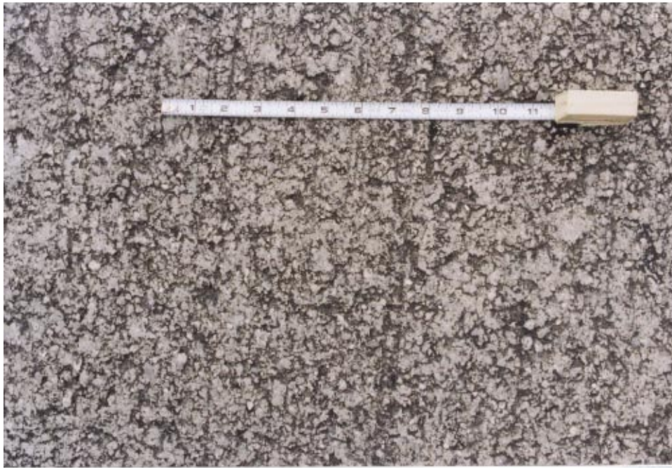
Figure 44 Typical RCC pavement surface at the GM Saturn plant.
