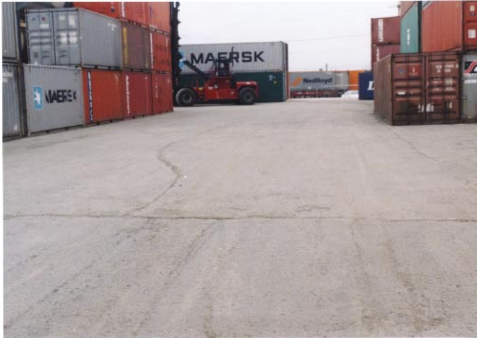
Figure 17 Conley Terminal, Boston, MA. Built 1986.
